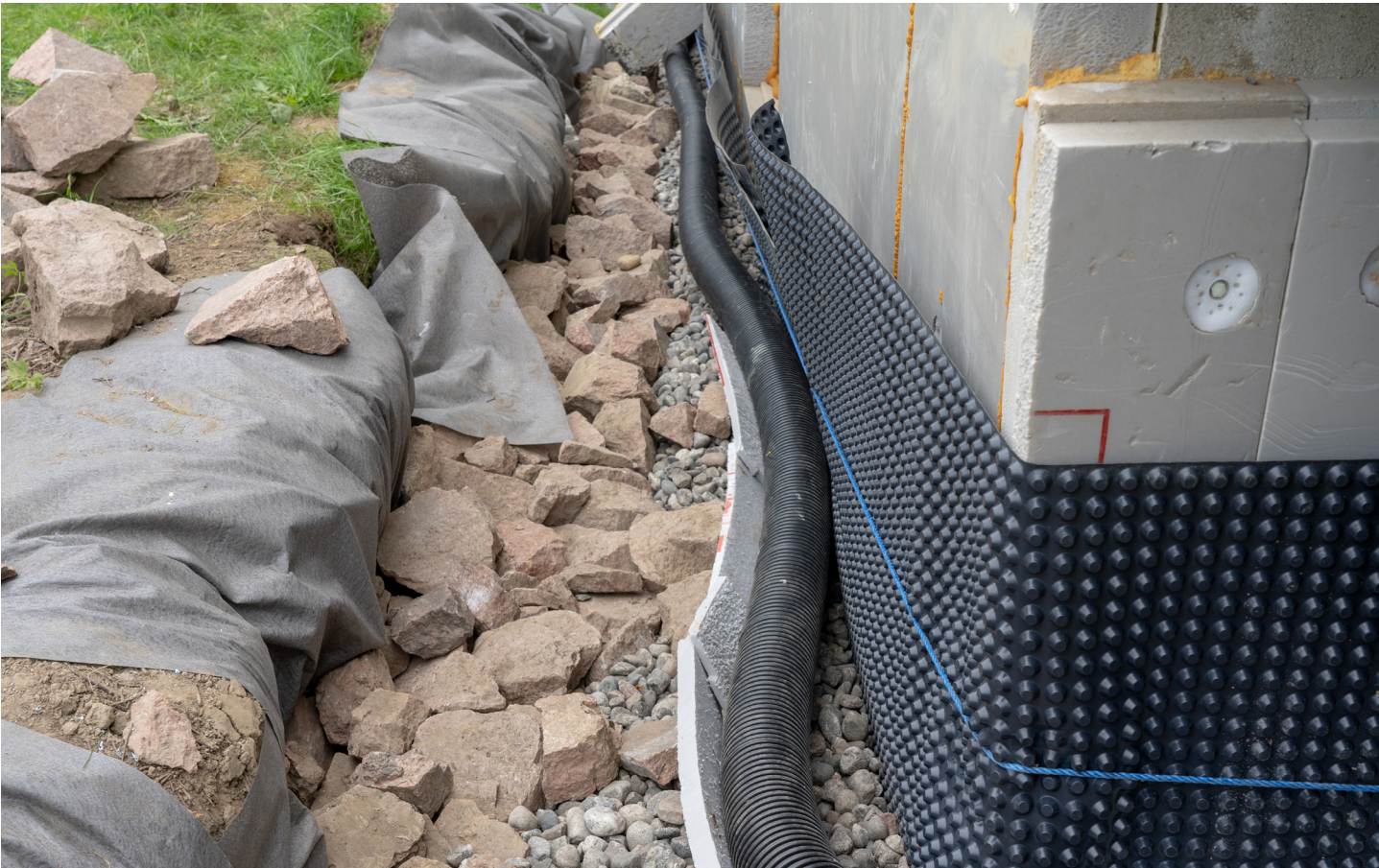
Drain tile installation on the exterior of home footings. Read more: Office of Energy Efficiency & Renewable Energy: Footing Drain Pipe
