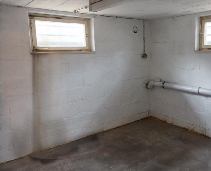
Unaddressed basement window seepage can lead to standing water, damp and humid air, order, mold and mildew.
